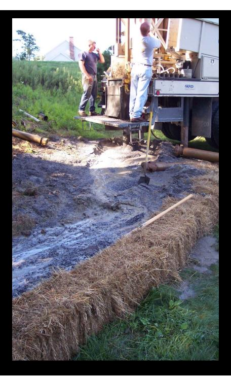
Straw bales keep well drilling slurry and rock fragments from spreading over existing landscape
