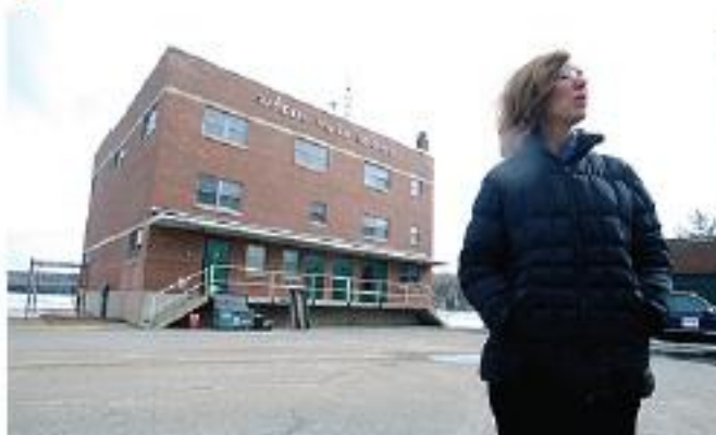
Kathy Moriarty General Manager of the Bangor Water District at the Floods Pond pumping station in Otis. The Bangor Water District pumps about 5 million gallons of water per day. The drinking water is periodically tested for over 200 contaminants and is also treated at a separate facility before entering the water supply. (Bangor Daily News/Gabor Degre) Buy this photo
