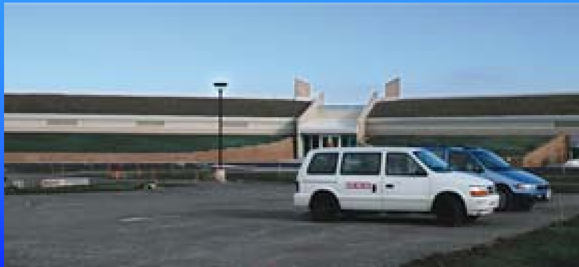
Permeable Parking Area
