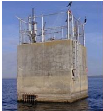
Surface Water Intake
