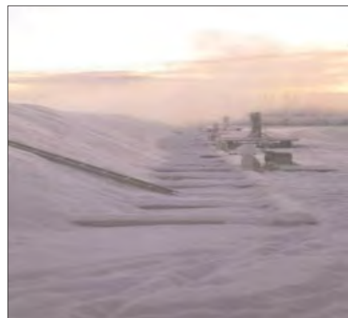
Defying the Odds In Fairbanks, Alaska, the composting operation at a wastewater treatment plant goes on year-round, silencing skeptics who weren't convinced the process would generate enough heat to kill pathogenic bacteria during the extremely cold winter months.
