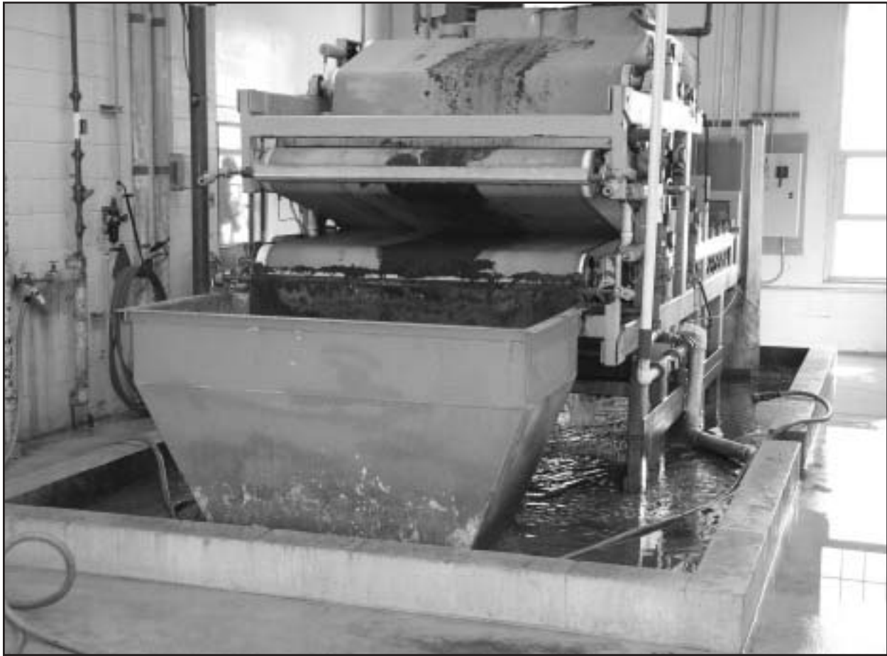
When sludge is dewatered with a belt filter press, samples should be collected as the material exits the press. Note the accessibility issues and potential safety hazards present.
