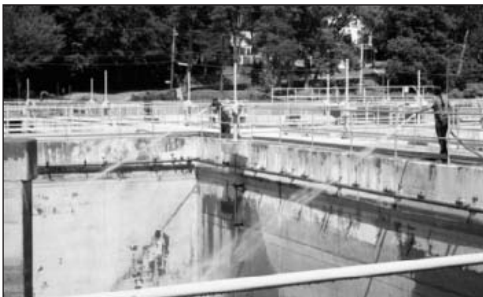
Lowell Wastewater Treatment Facility.
