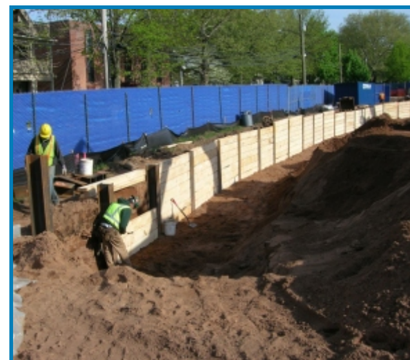
Sediment & erosion controls/shoring.
