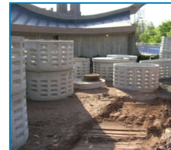
Groundwater recharge drywells.
